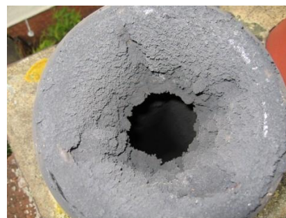
Figure 14 - Chimney sweeping annulus
