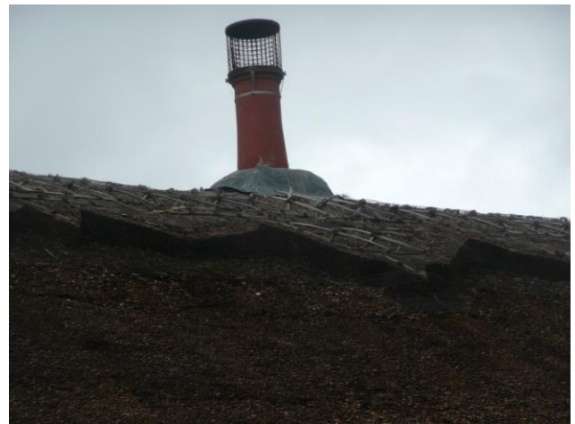
Figure 12 - Long-pot used to increase thatch to pot top clearance
