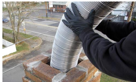
Figure 9 – Flexible lined chimney
