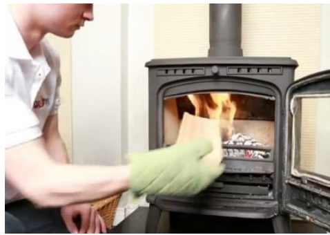
Figure 6 - Example of multi-fuel stove with single door providing access for fuel loading and ash-pan removal
